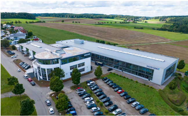
The company headquarters of montratec GmbH in Dauchingen (Germany).
